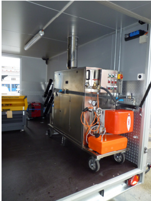
The steam generator installed mobile...
